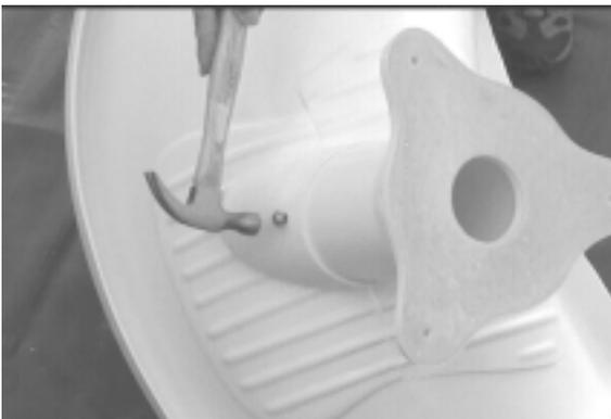
2. Using the 1" long bolt and corresponding washer, insert 3/16" roll pin onto bolt. Use a hammer to gently tap the bolt assembly into the pipe/receptor.
