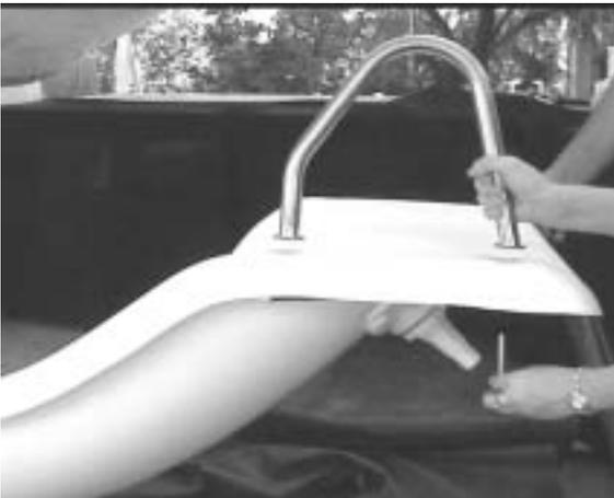
3. Lift the flume up to its upright finished position and align the holes of the rail underneath the holes in the seat area of the flume. Use 3/8" X 3" bolts with washer inserted from the bottom up to attach rail to flume and to the grab rail placed on top of the flume holes. Note: Straight to bend portion of the grab rail is closest to the ladder end. The angle bend is closest to the flume. Secure with a 9/16" wrench.
